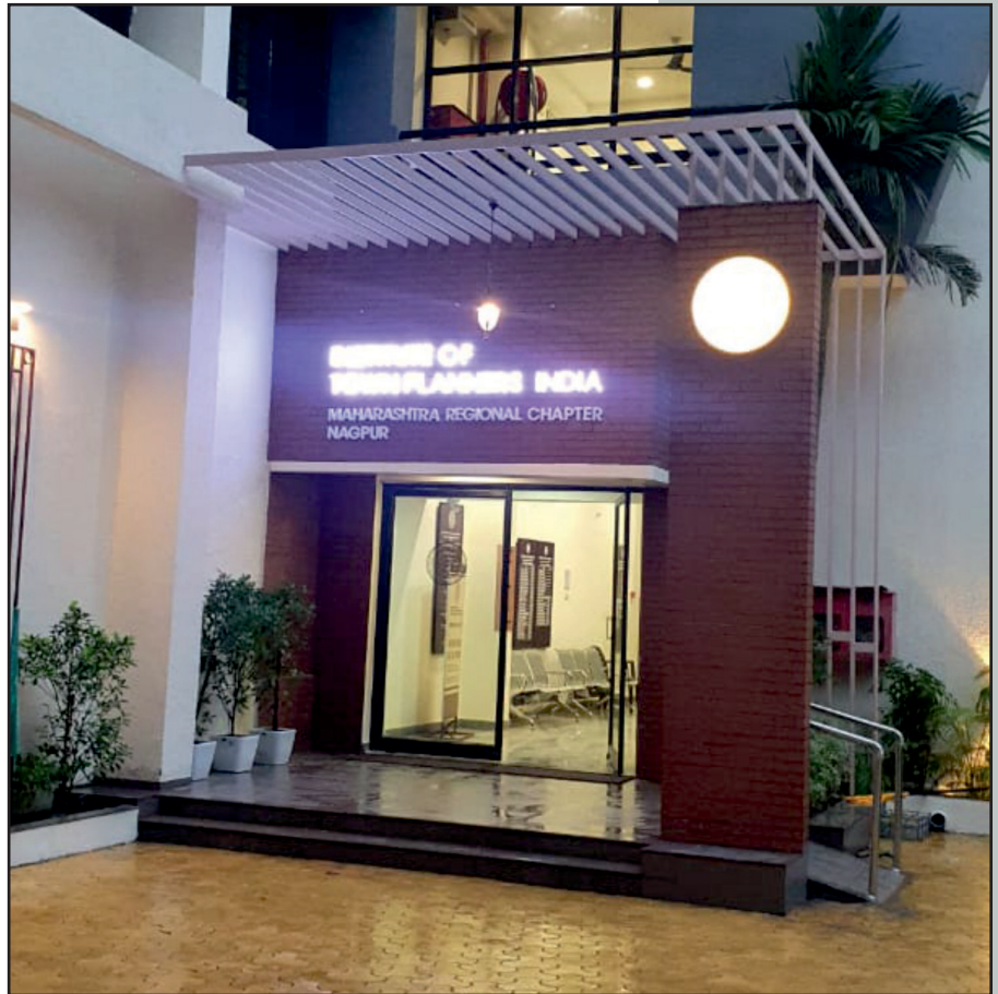
Entrance view of newly renovated MRC (N) Building
