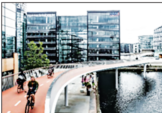
Fig. 5: Copenhagen Bicycle Bridge
