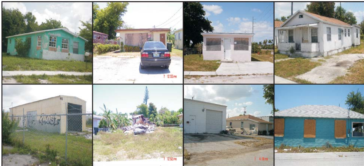
Fig. 4 The Condition of the Slum / Blight Areas
