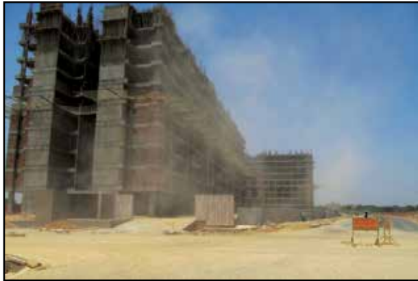
Fig. 8: Dust Cloud due to Construction Activities at Apple Wood Township
