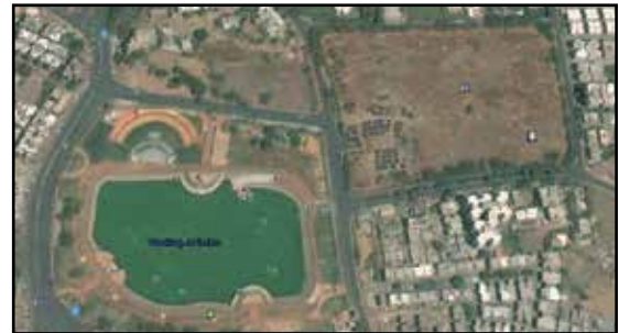
Fig. 10: Pre-project Site Conditions
