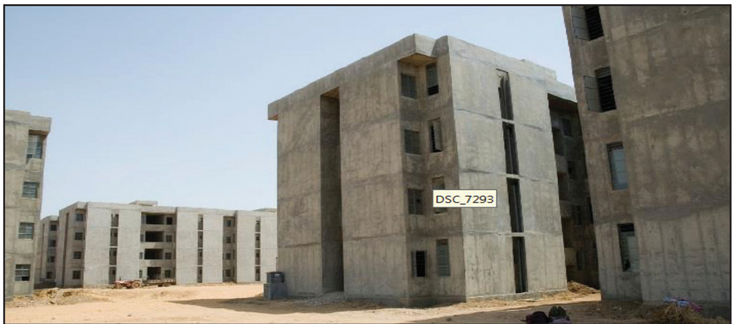
Fig. 10 (c) : View of Prahaldnagar TPS
