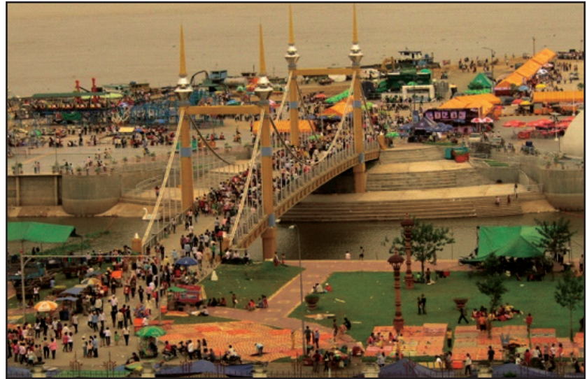
Fig. 6: Koh Pich Bridge before the Tragedy (Chanbo)
